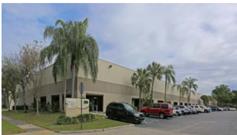
BUILDING 2000 16,908 SF AVAILABLE
